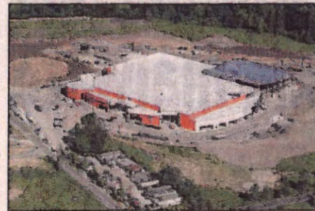
The casino takes shape as construction continues in May 2016.
