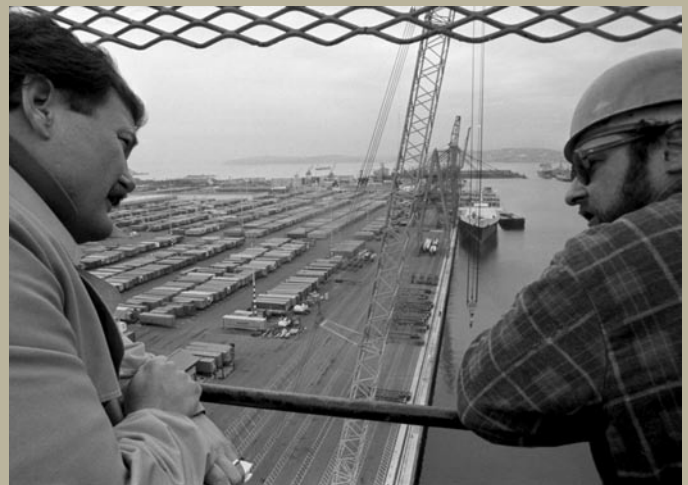
Men looking out over Port Of Seattle docks in January 1987
