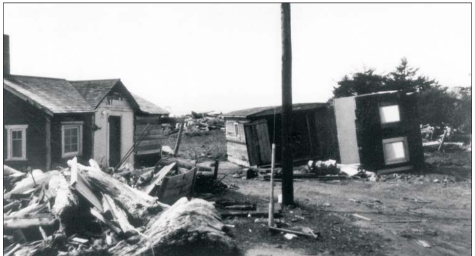
Figure 5. Photo 8-2-A. Portion of house completely torn from main part. Entire house was moved northwest 40 ft (12.2 m) from foundation. Map location 9.
