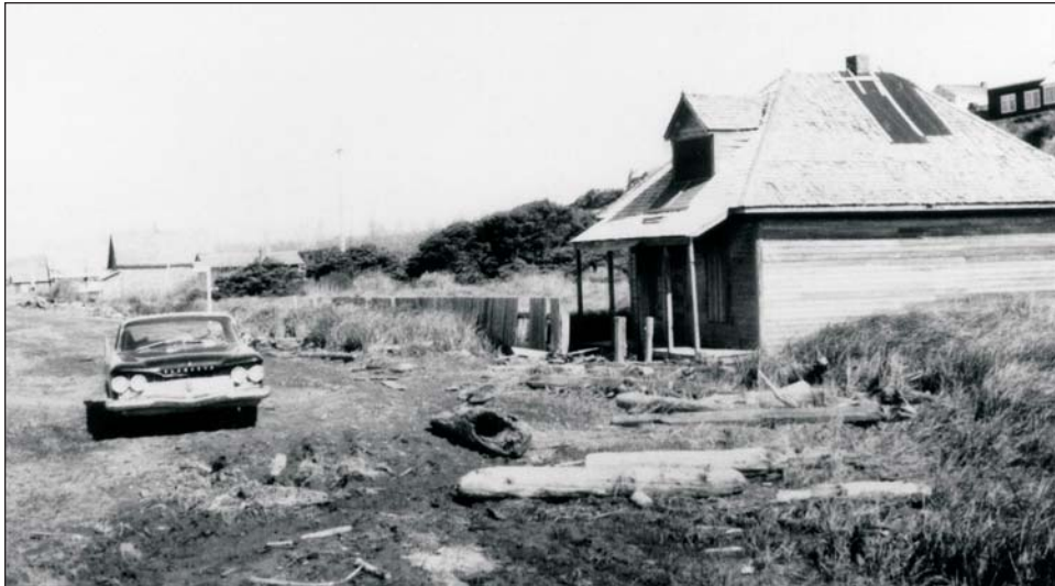
Figure 6. Photo 8-1-A showing drift line. Slough in back of house with debris scattered showing evidence of backwater. Map location 10.
