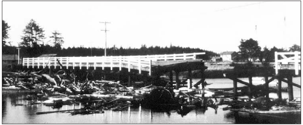
Figure 3. Photo 9-1-A. Two spans lost and timber bent. Two other 20-foot spans are shown considerably deflected. Map location 5.
