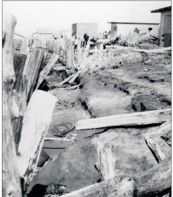
Figure 8. Photo 8-1-C showing erosion of bank and damage to bulkhead. Map location 10.
