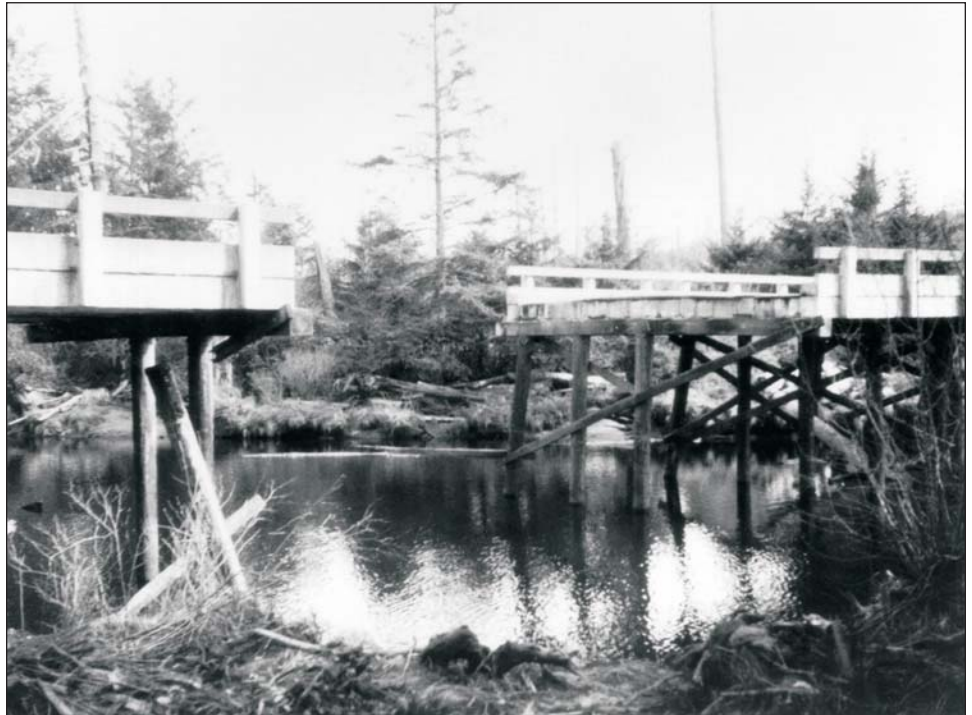
Figure 4. Photo 8-3-A. Two spans of bridge and middle pile bent lost. Pile bents on each side damaged, right side has been deflected from original position. Map location 8.
