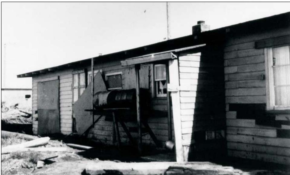
Figure 7. Photo 8-1-B showing windows broken, siding torn off, and drift logs scattered in back yard. Map location 10.
